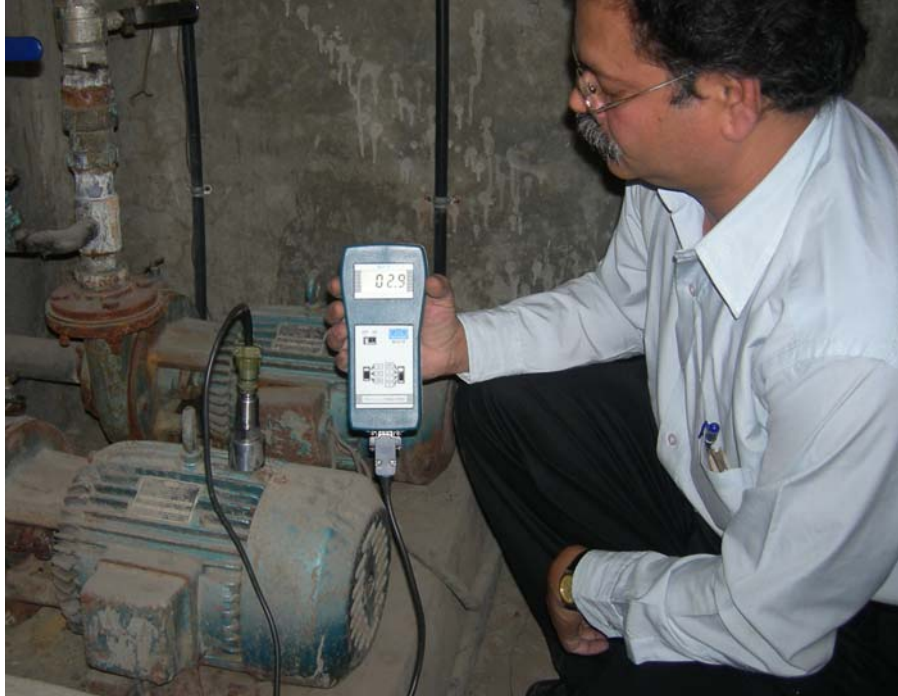
Figure 1 Periodic Vibration measurements save valuable machine downtime
