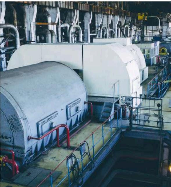
Our Online Systems IRD7100 MPT as well as IRD8800 MPS API670 also come for Turbine Supervisory Instrumentation (TSI). Parameters such as Vibration, Temperature, Speed, Differential Expansion, Casing Expansion, Cam Valve Position, Axial Gap, Eccentricity and more are monitored on a Continuous basis to protect Turbines and Generators that are critical and could be producing any amount of power from 5 MW, 210 MW, 500 MW, 660 MW, 800 MW or more.
