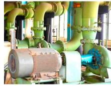
A pumps power consumption often accounts for over 12% of the total electricity used and it is a well recorded fact that an out of balance rotor will consume or waste up to 15% more energy.
